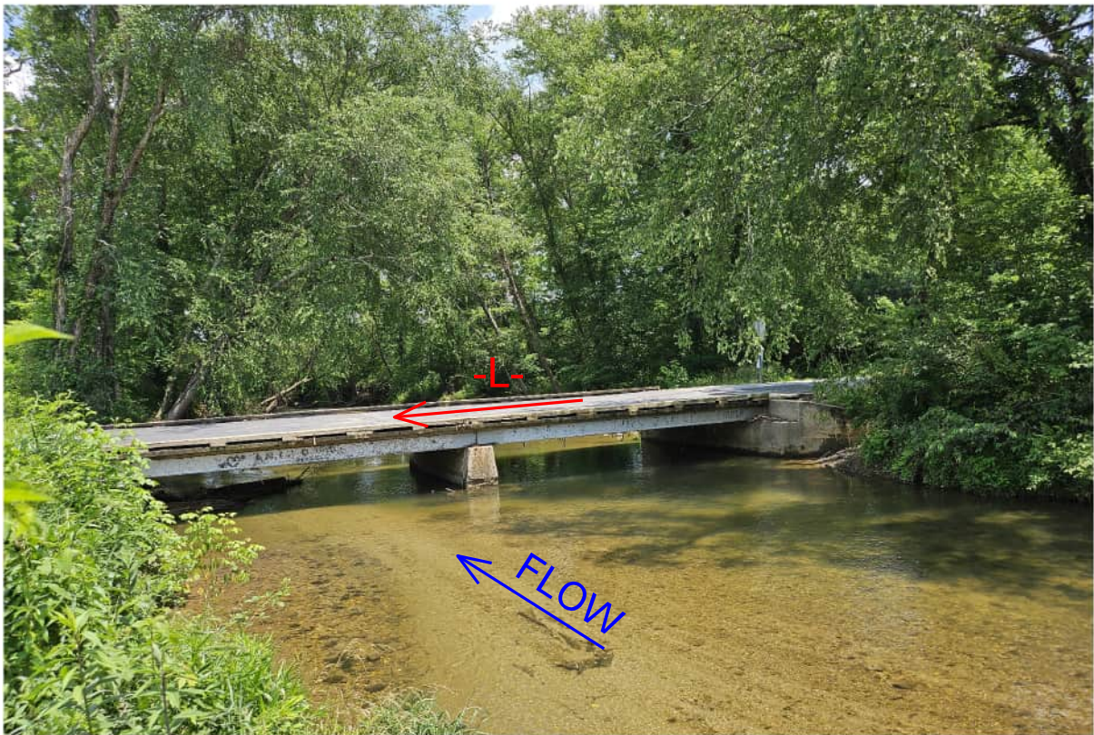
NORTH WEST SIDE BRIDGE LOOKING DOWNSTREAM
