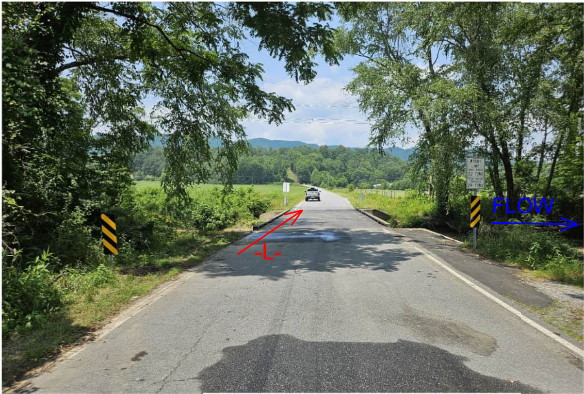
SOUTH APPROACH LOOKING NORTH ALONG -L- ALIGNMENT
