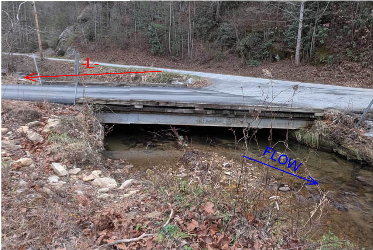
WEST SIDE BRIDGE LOOKING EAST (UPSTREAM)
