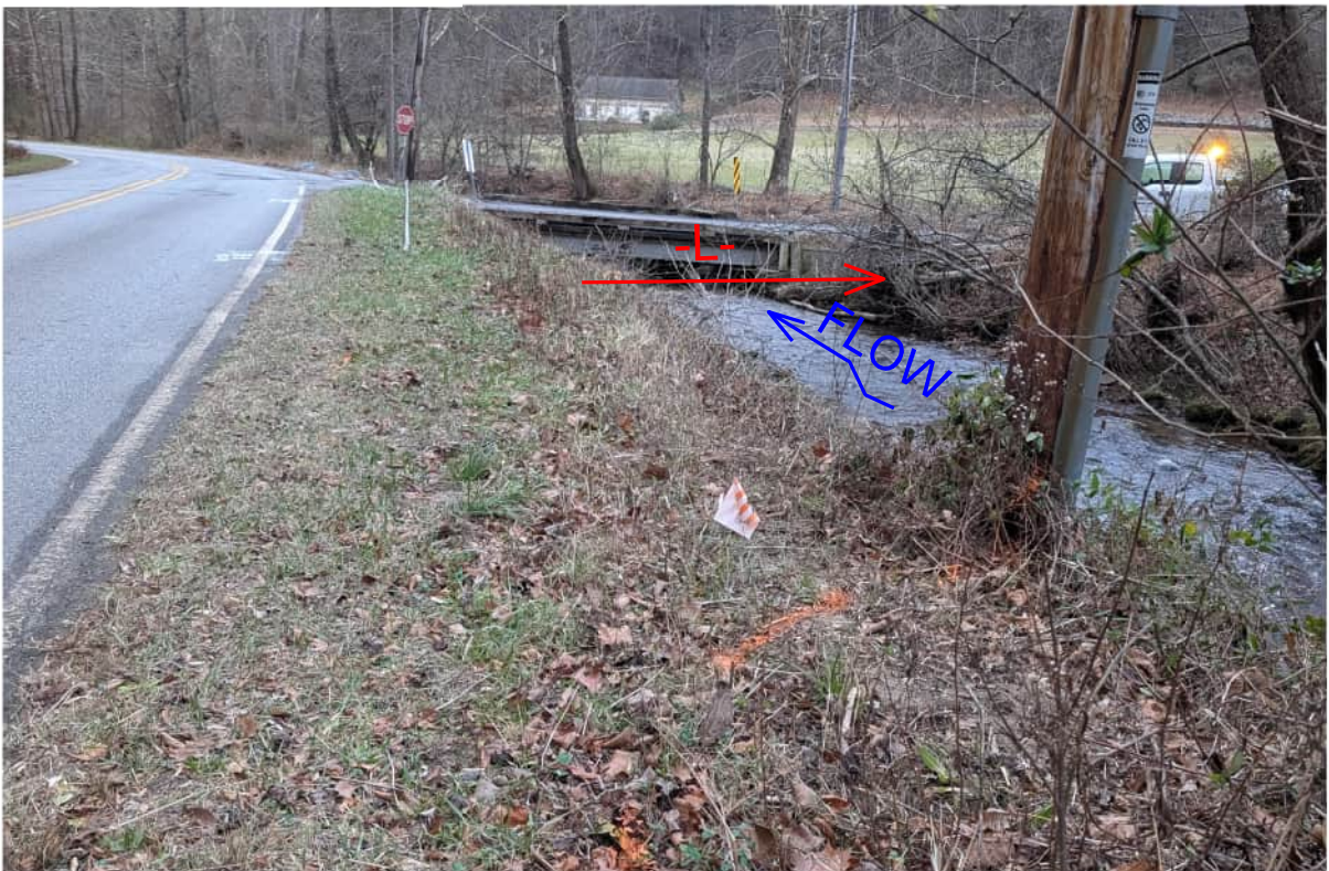
EAST SIDE BRIDGE LOOKING WEST (DOWNSTREAM)
