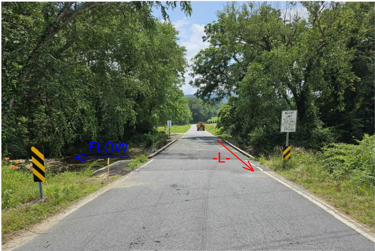
NORTH APPROACH LOOKING SOUTH ALONG -L- ALIGNMENT
